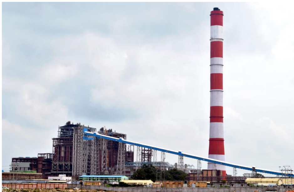
Image: 2x500 MW Koderma Thermal Power Station
